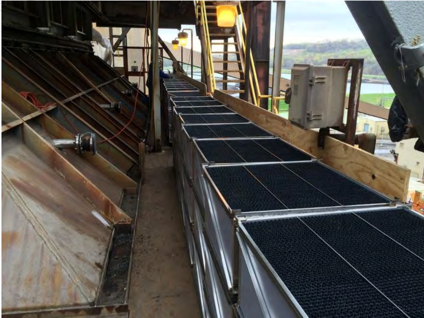
Modules Staged at Elevation, Ready for Installation
